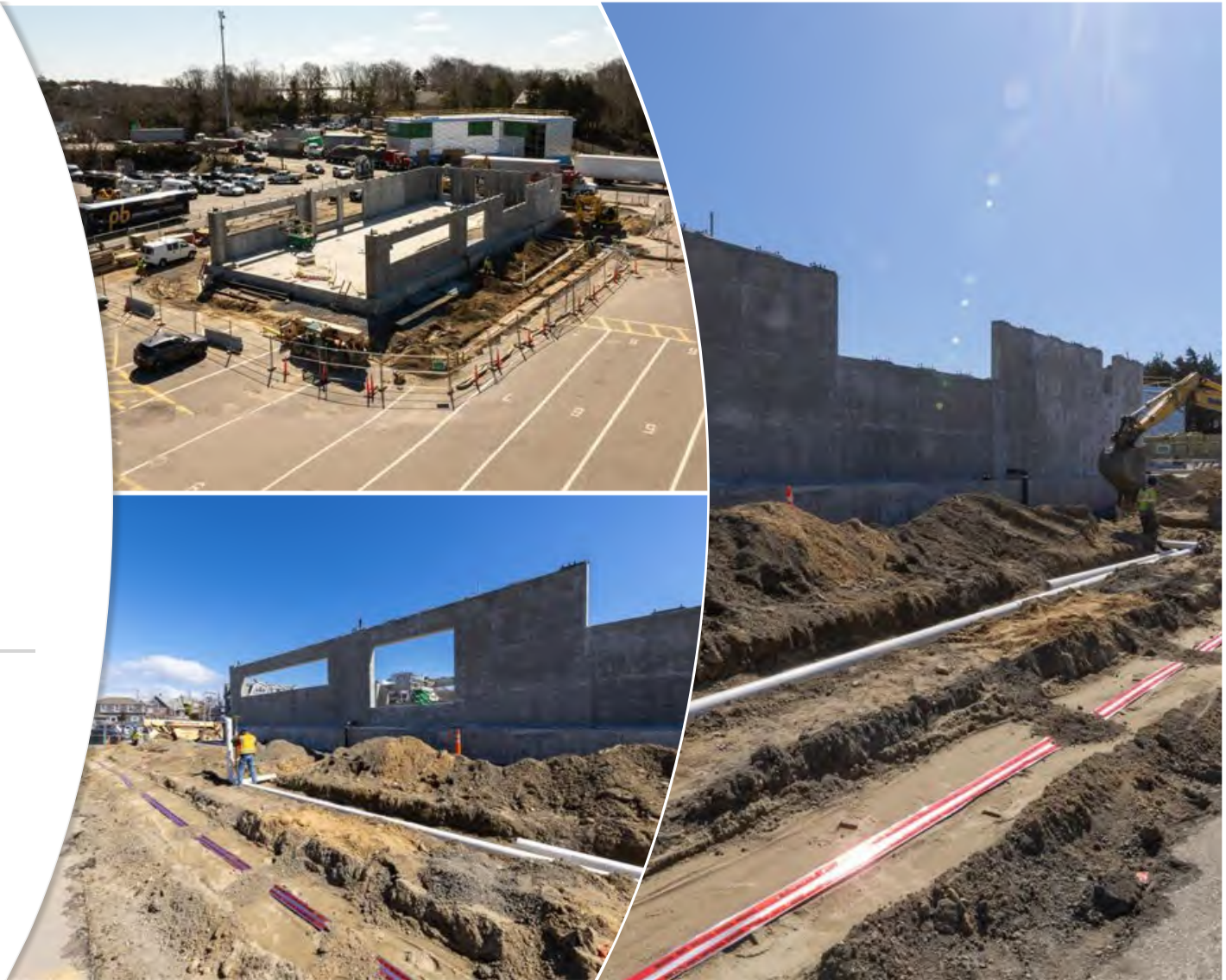
Installation of perimeter drainage at the Terminal Building
