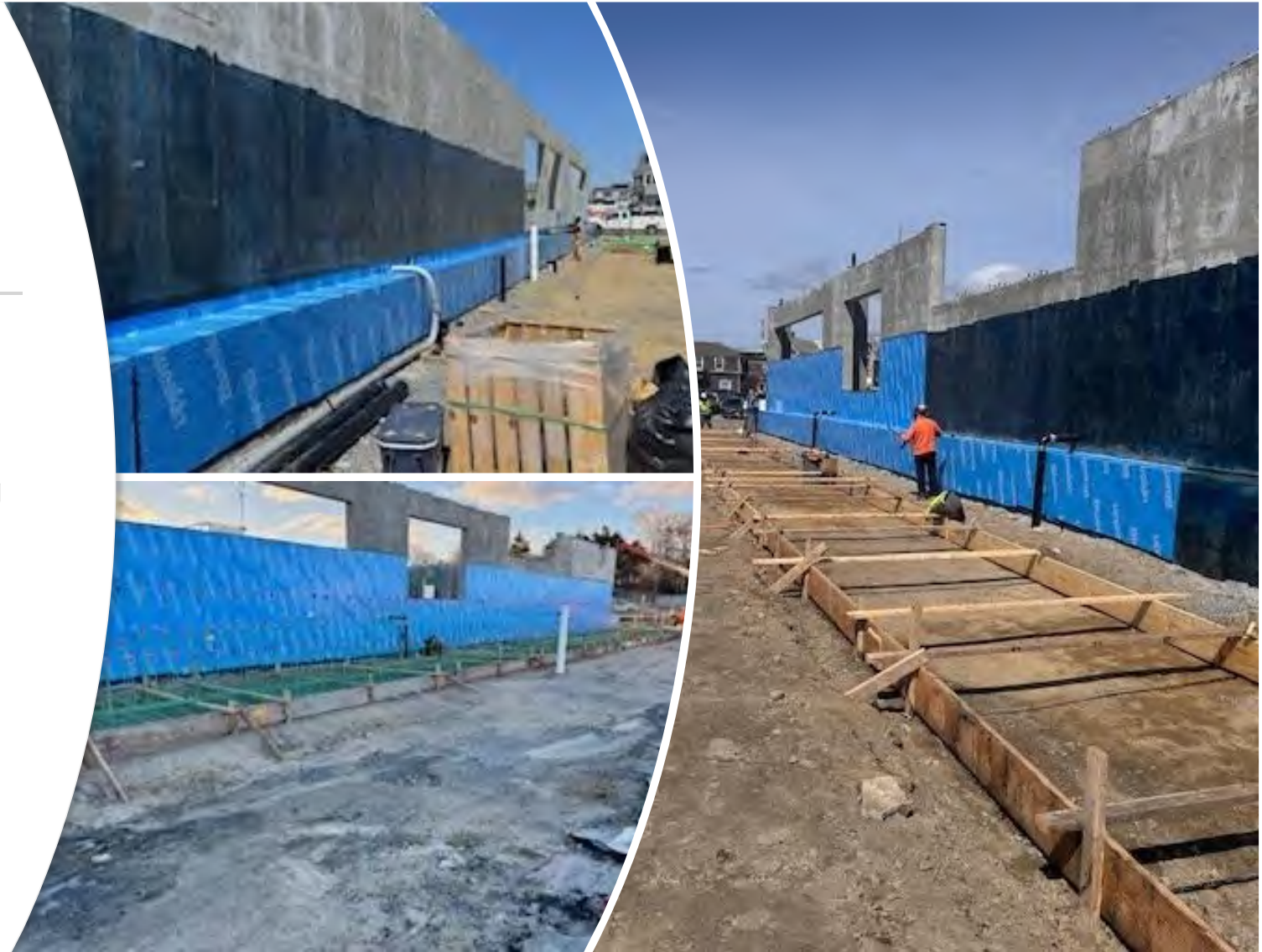
Waterproofing concrete wall at East and West side of Terminal Building
