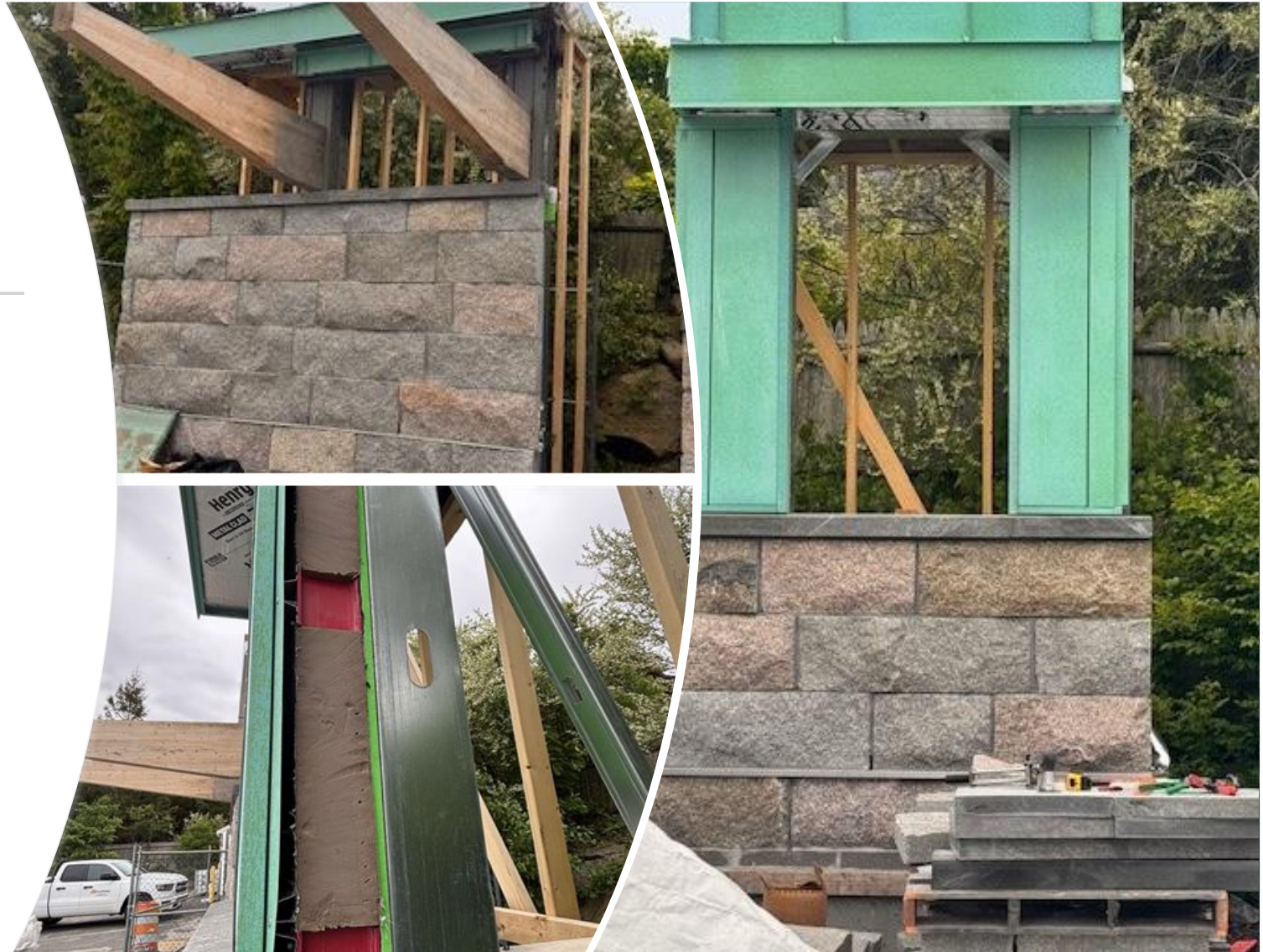
Mock-ups of the Terminal Building and Utility Building with the copper clad siding for testing and performance
