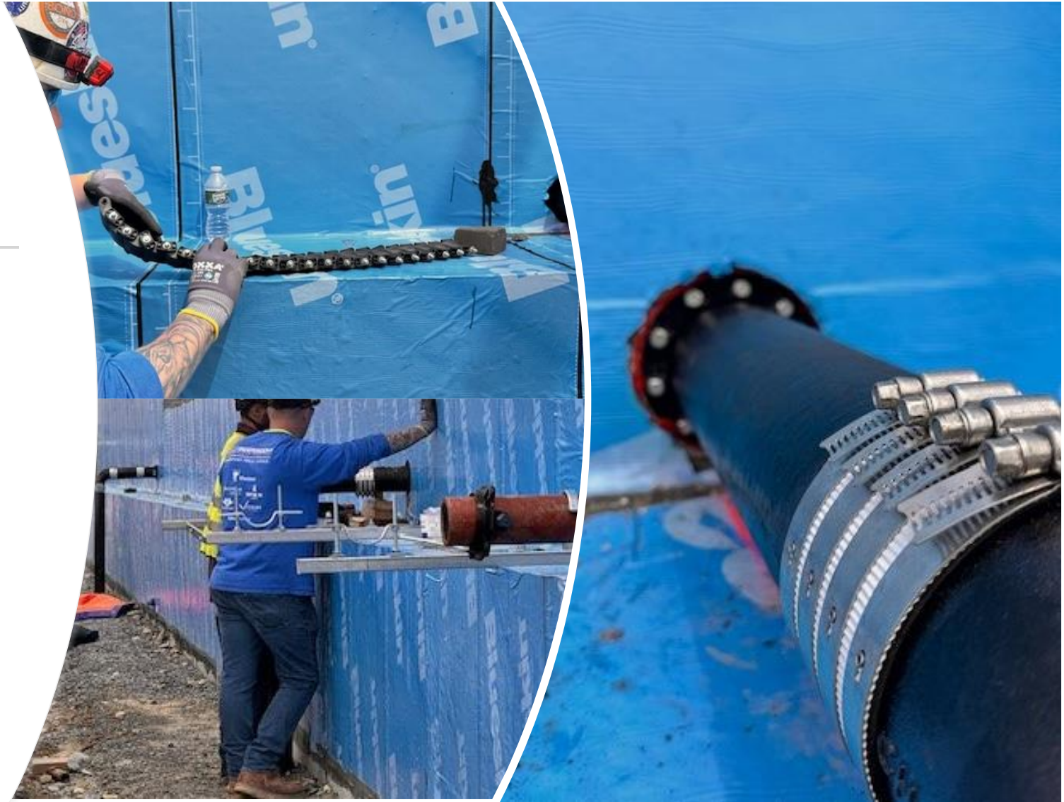
Installing rubber pipe insulation to all drainpipes at the Terminal Building
