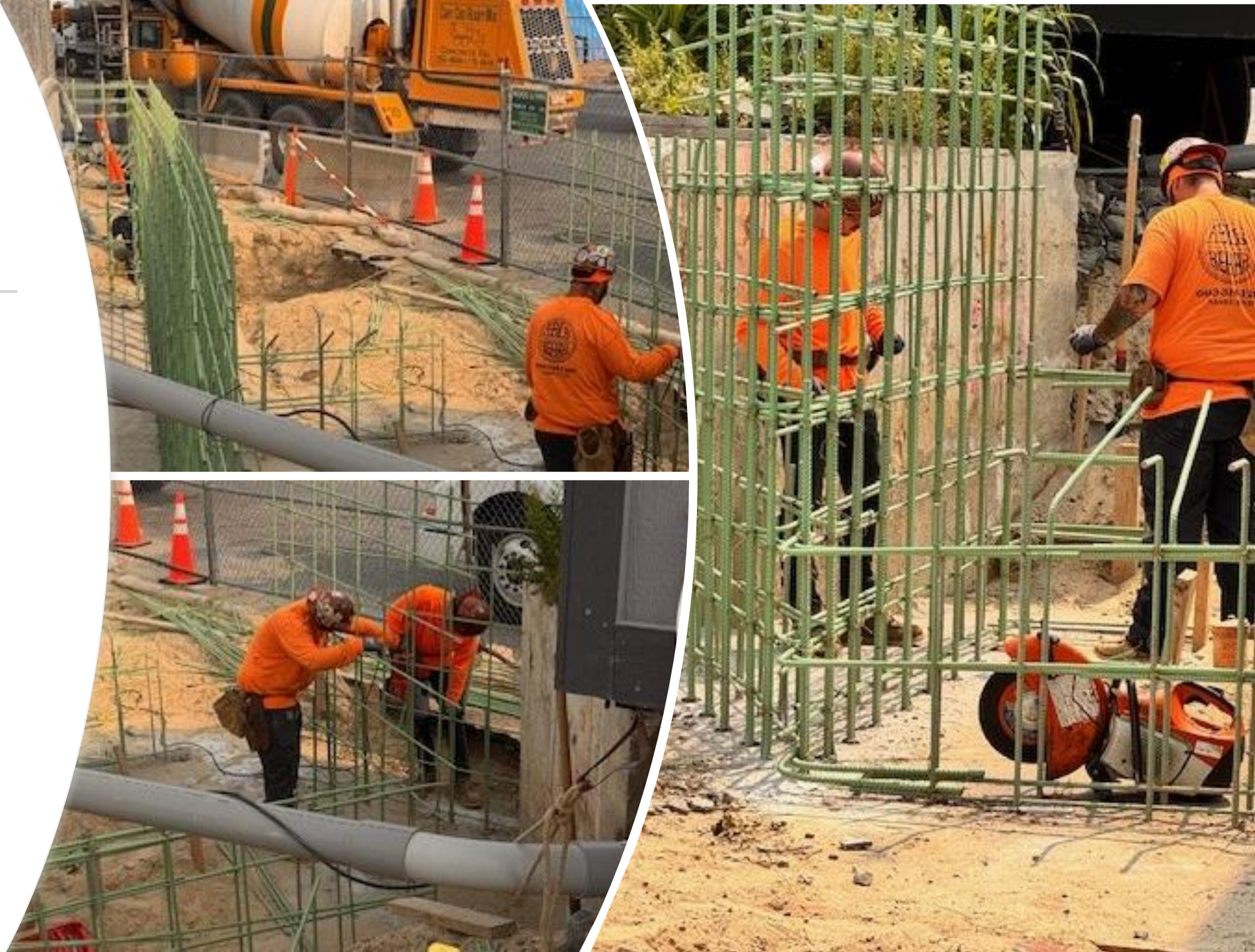
Installation of rebar at stairwell #2 wall and footing at the Utility Building
