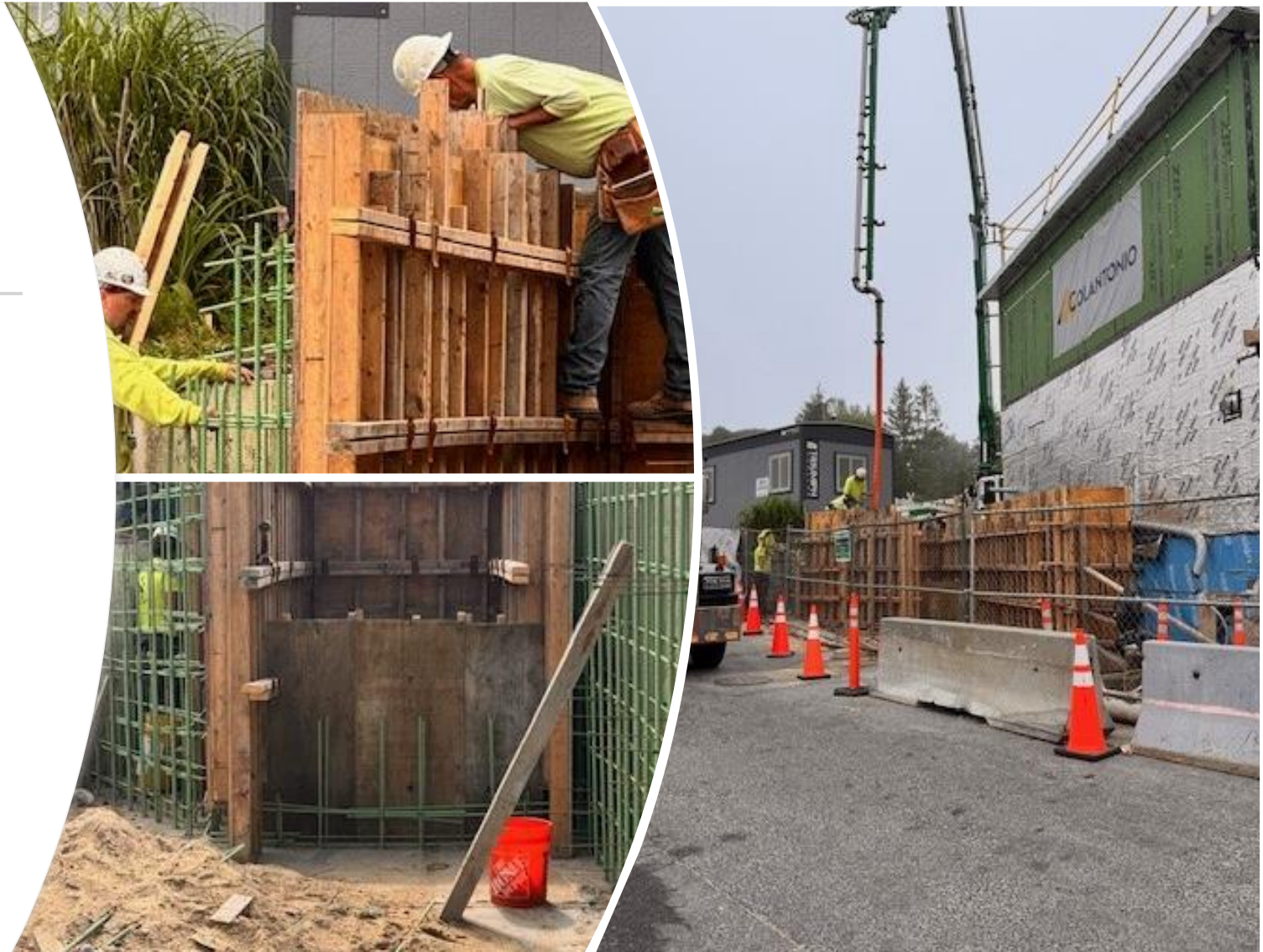
Installation of retaining wall and footing forms and concrete pour for the stairwell at the Northeast corner of the Utility Building
