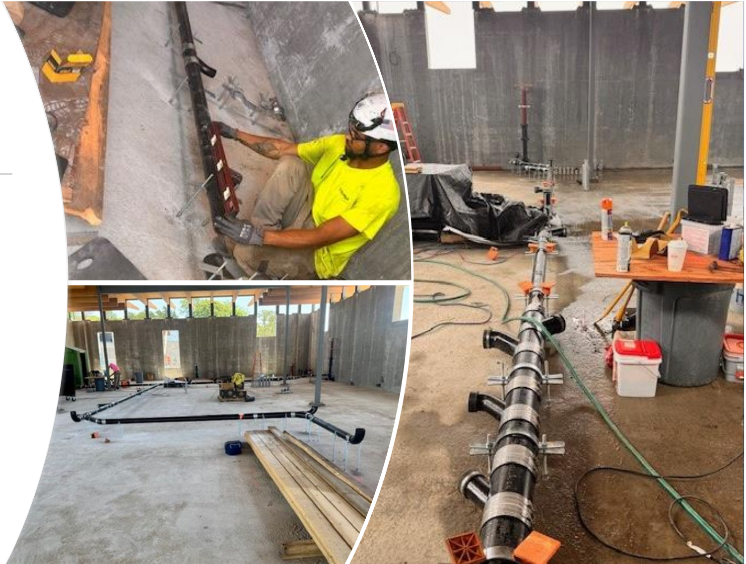
Plumbers installing sub floor sanitary drainage lines for the restrooms at the Terminal Building.
