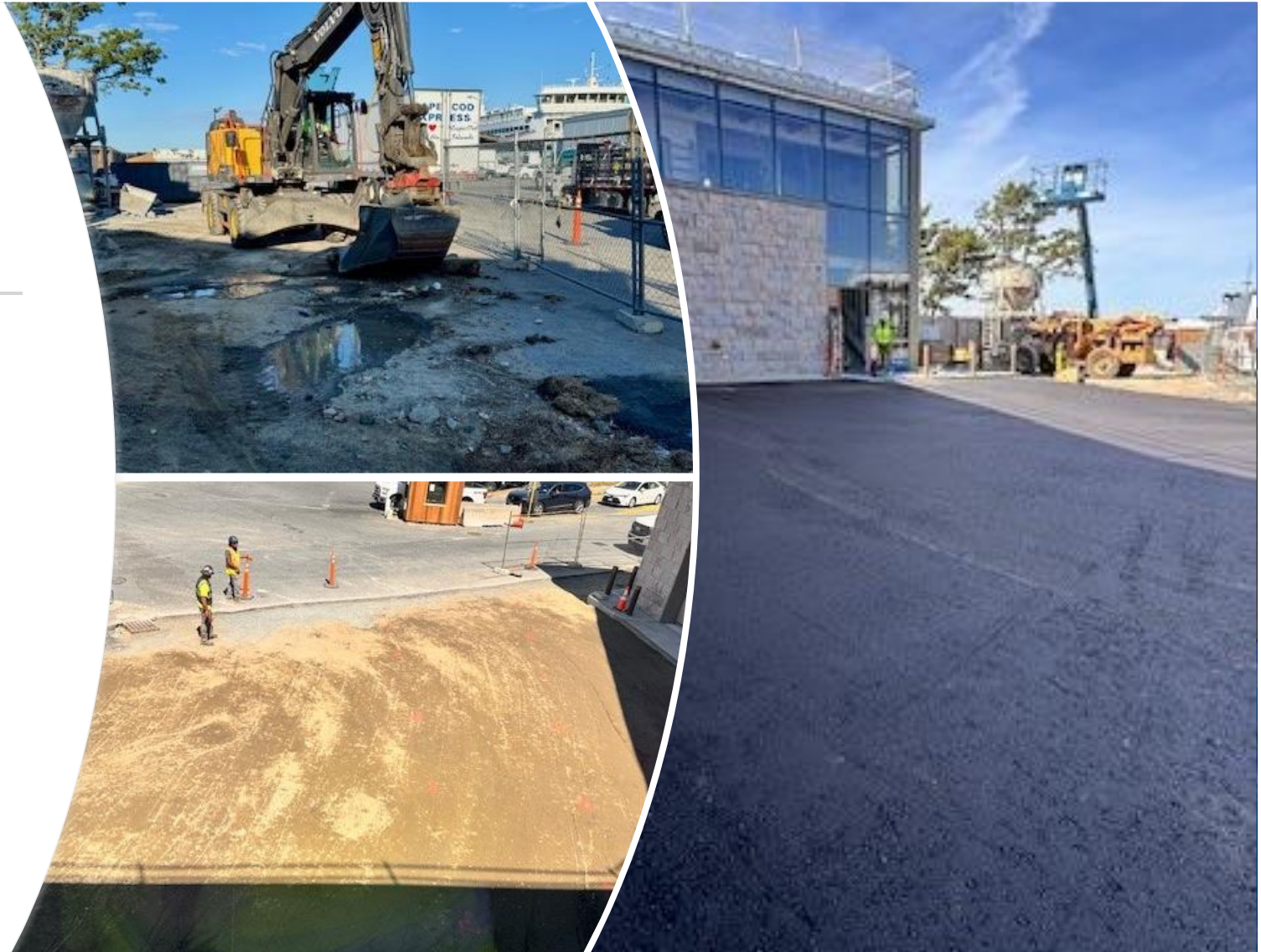
Re-grading and surface coating with pavement at the North Side of the Utility Building
