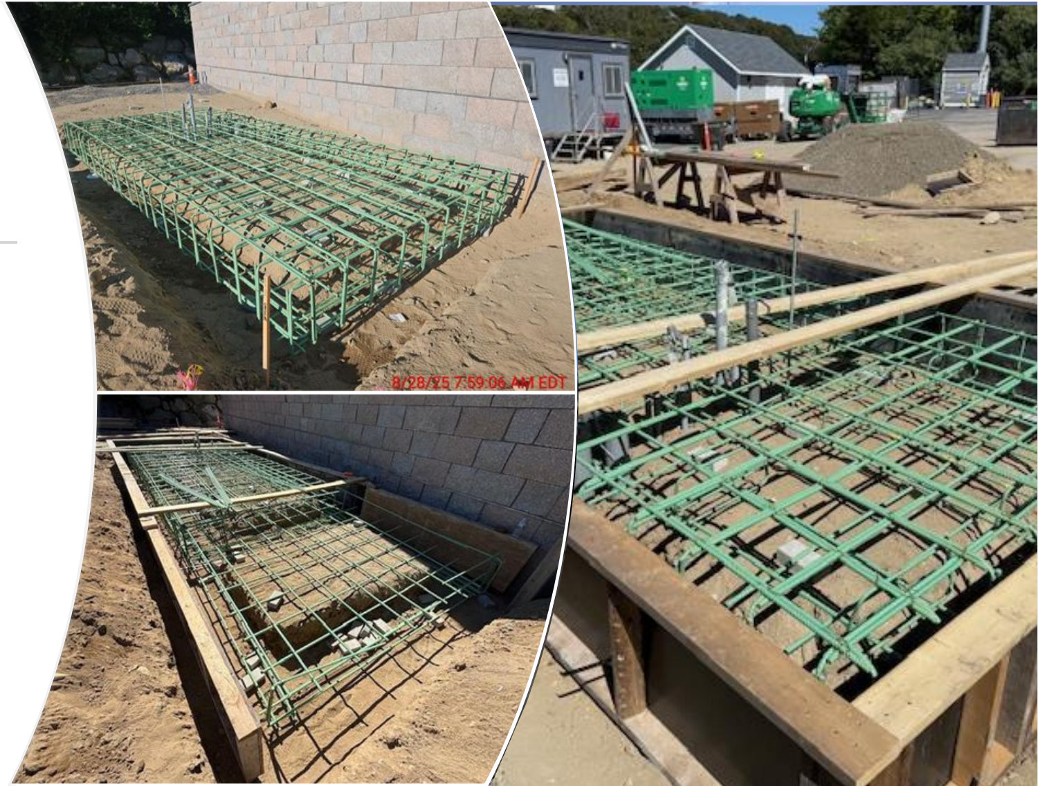
Rebar and form work to pour concrete for the generator pad at the East side of the Utility Building
