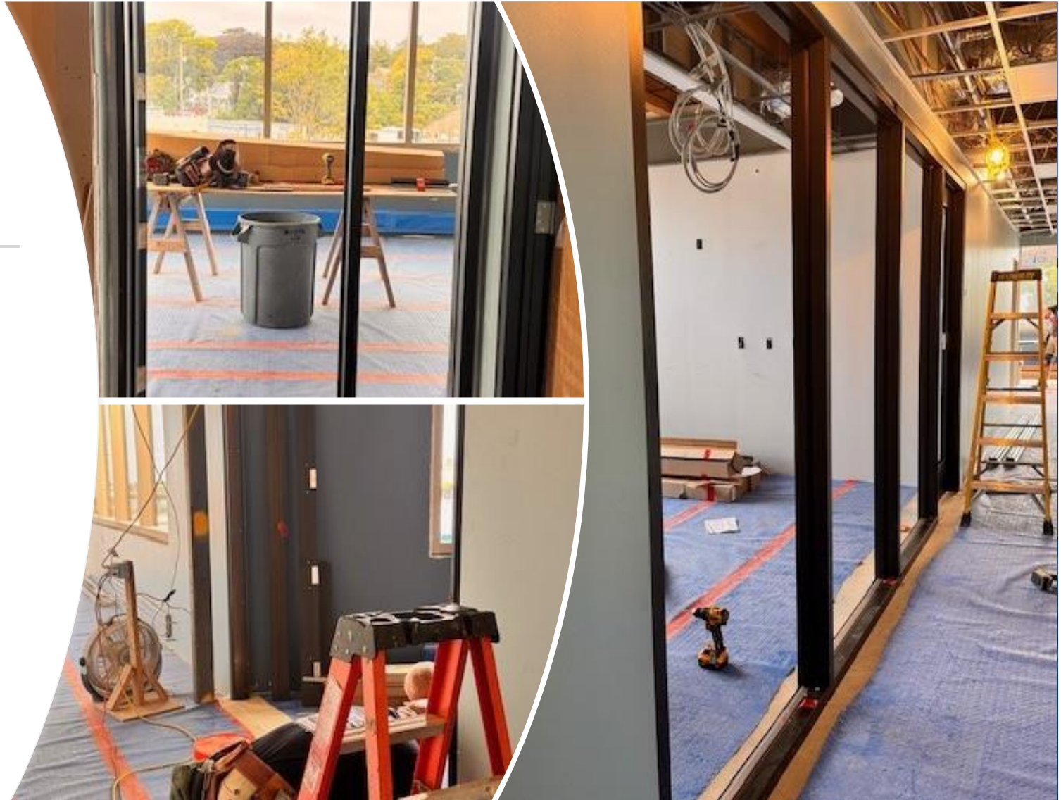
Carpenters install aluminum door frames at the Utility Building second floor.
