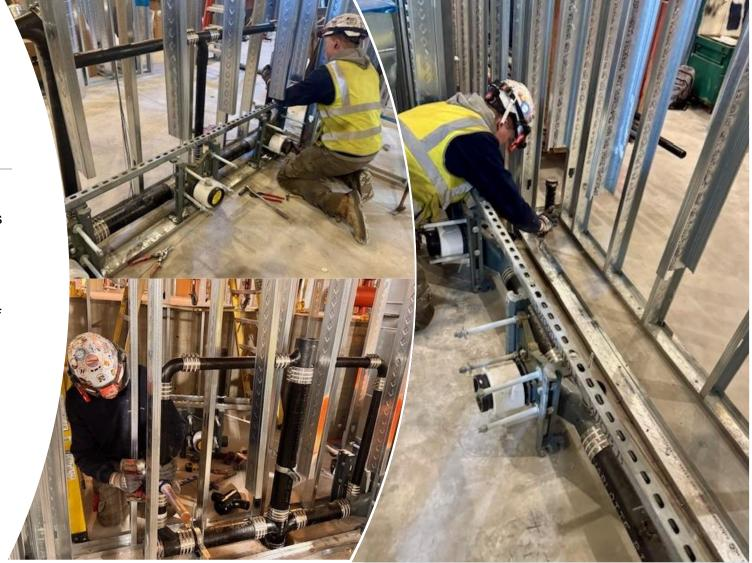
Pipe fitters install copper water lines to the geothermal manifold at the Utility Building.
