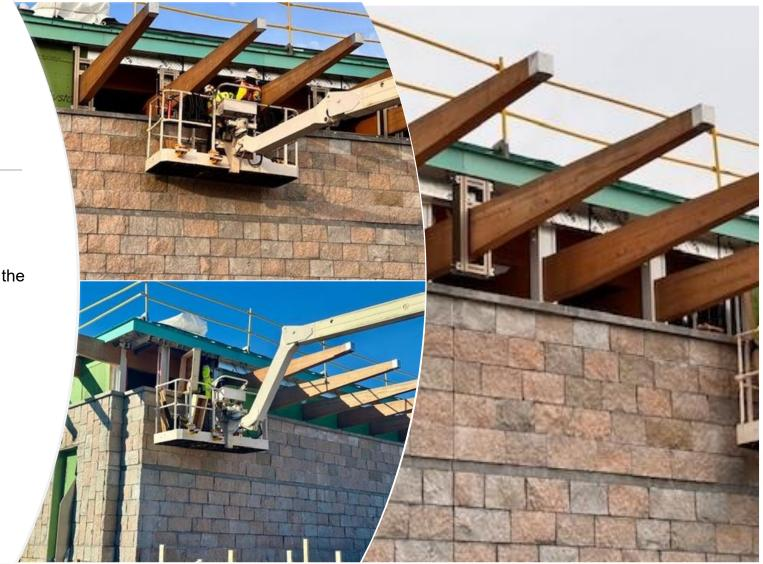
Window (curtain wall) brackets are installed on the East side of the Terminal Building
