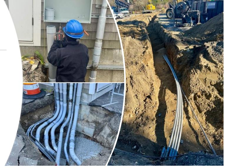
Electricians install conduit lines for making connections from the electrical shed to the Utility Building for Data and Communications.
