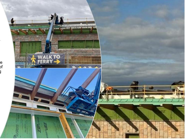
Copper soffits and fascia are being installed on all sides of the Terminal Building during all kinds of weather.
