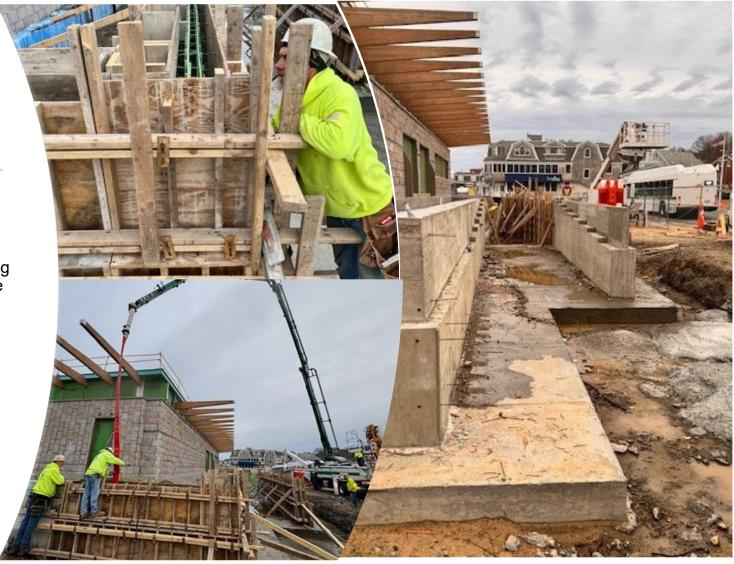
The formed retaining walls are filled with concrete and cured and shows the making of the stairs that will provide access to the Terminal Building from the East.
