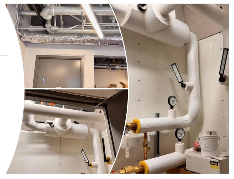
Pipe insulation is installed on copper water lines and air vents on the first floor of the Utility Building.
