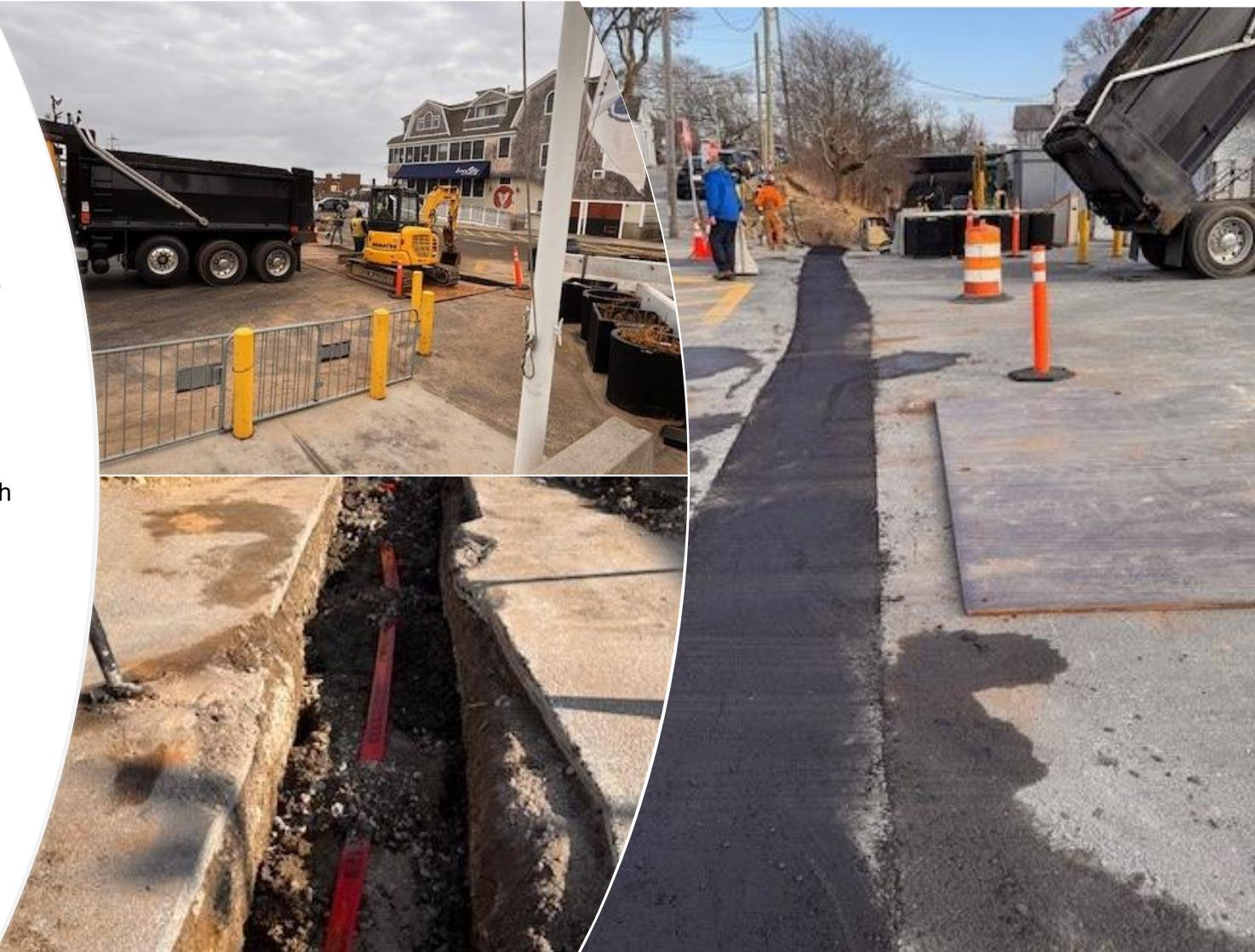
Electricians lay conduits for the Data lines that will connect from the Utility Pole through to the Data manhole, via electrical conduits, and back to the Utility Building and the Terminal Building.
