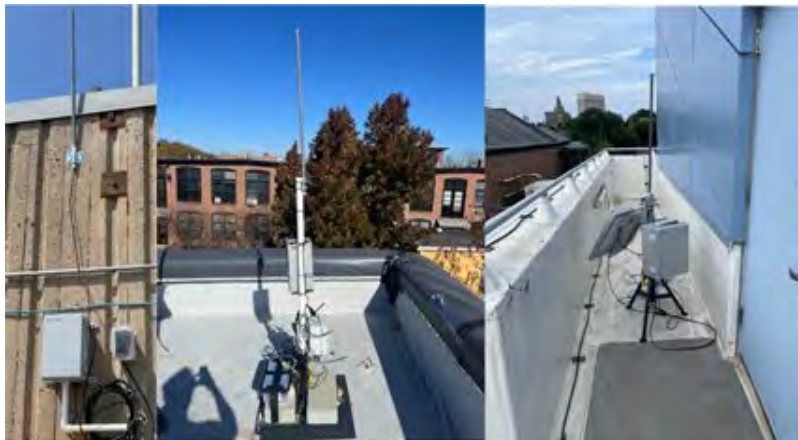
Figure 3: Example of gateway setups with hardwired power and internet (left), hardwired power and cellular internet (middle), solar power and cellular internet (right).
