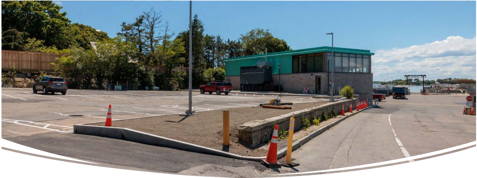
Woods Hole Utility Building
