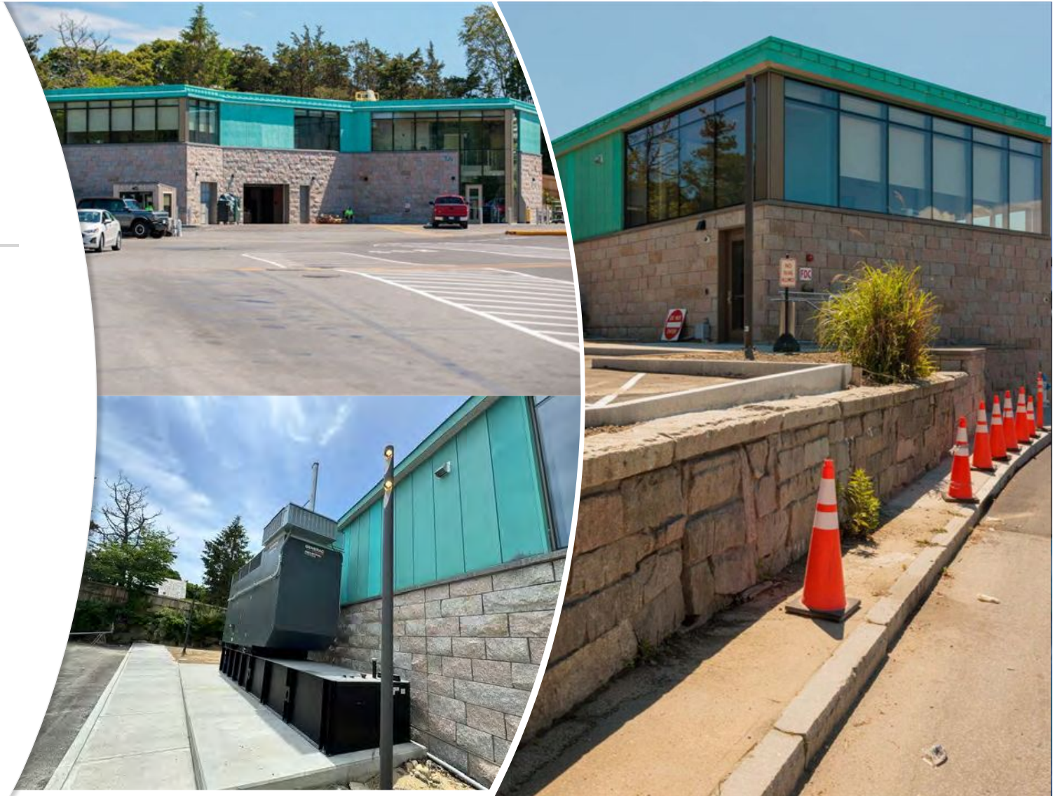
Utility Building Exterior
