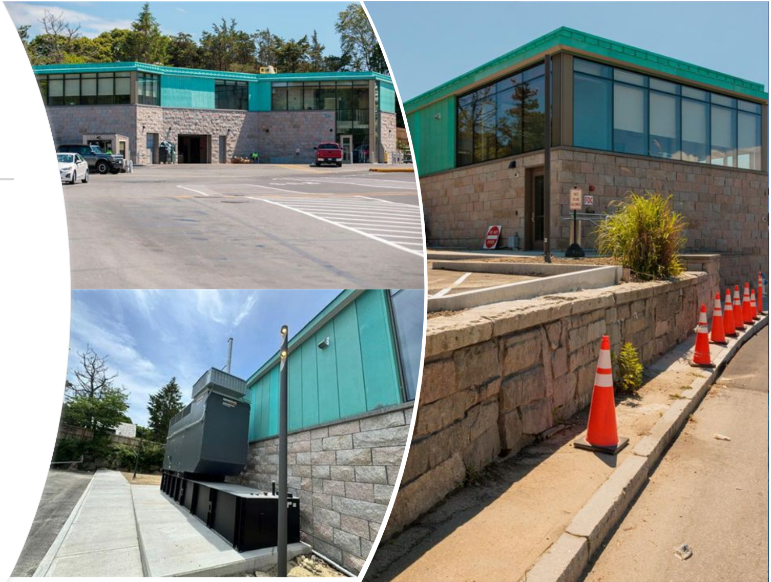
Utility Building Exterior
