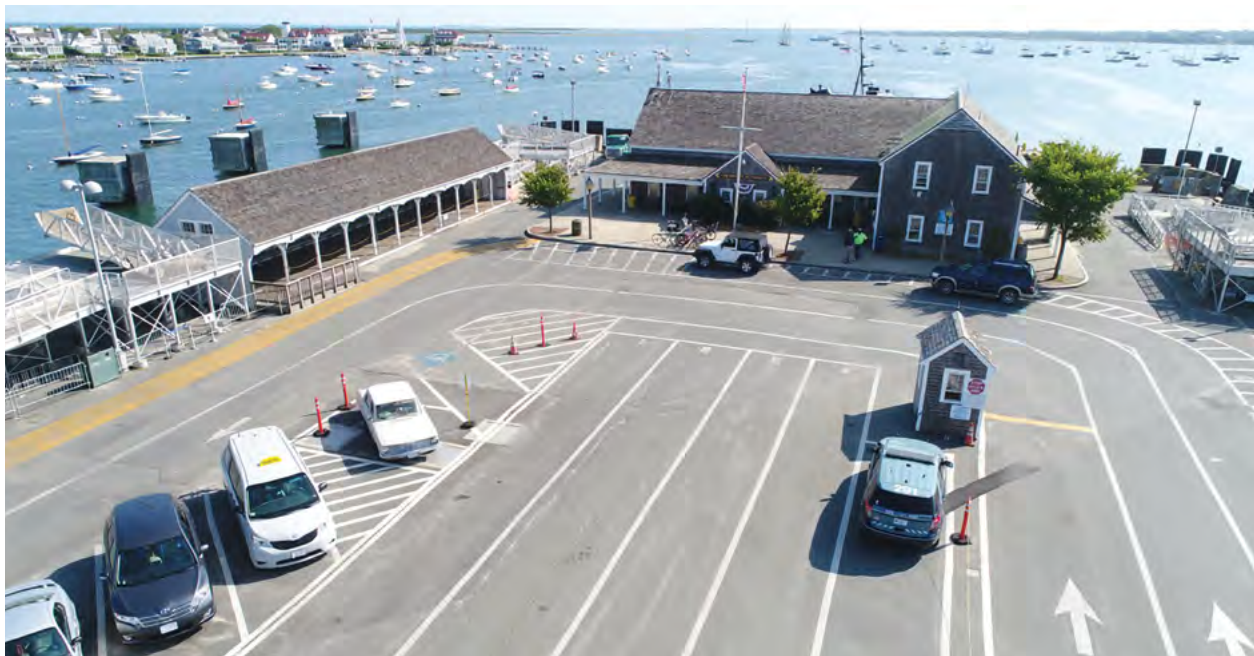
Aerial view of Nantucket Terminal.
